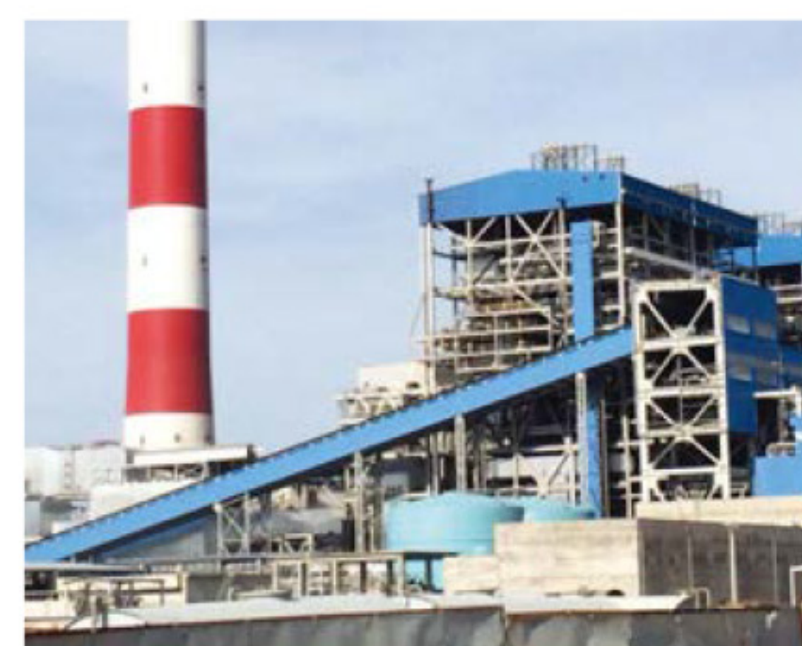
Vinh Tan Arch-Fired Units I & II Location : Binh Thuan Province, South Vietnam Customer : Vietnam Electricity (EVN) Start-Up Year : 2013 - 2014 Capacity : 2 x 622 MWe Fuel : Anthracite
